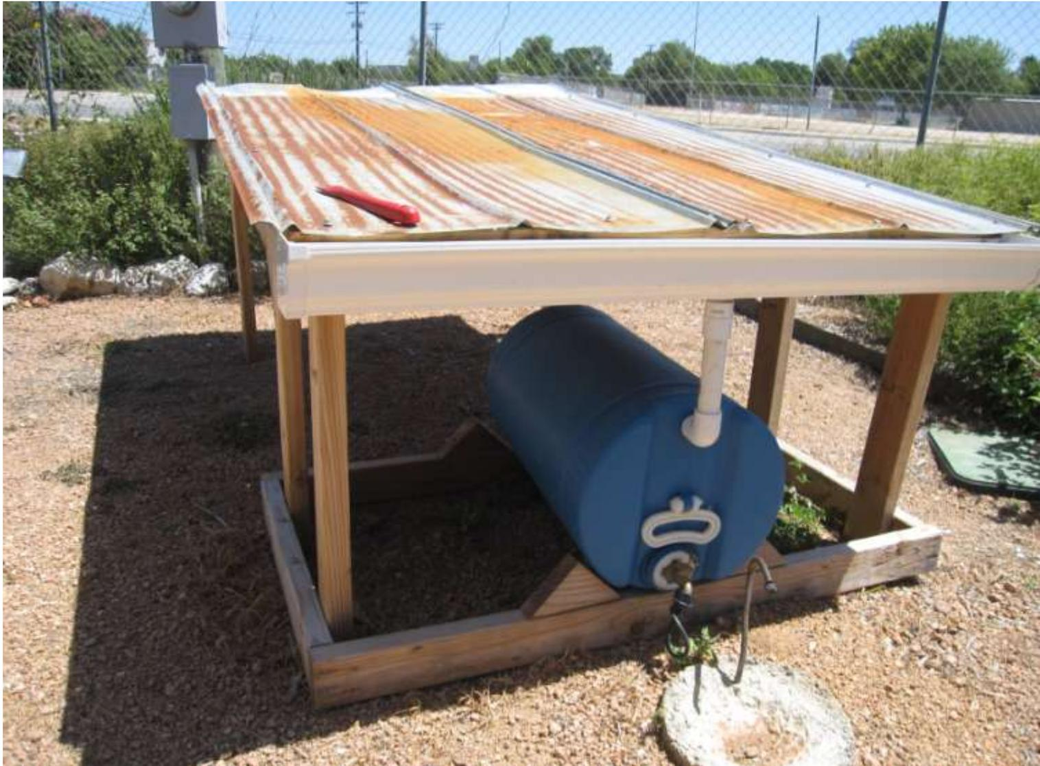
The Kerrville guzzler has a 30 gal barrel and is laying on its side. It requires a frame to support it and keep it from being jostled. This is a 7 ft long guzzler and made according to the “Original Diagram”
