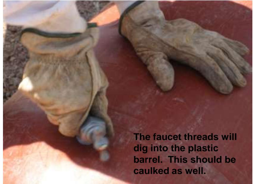
**The faucet threads will dig into the plastic barrel. This should be caulked as well.**
