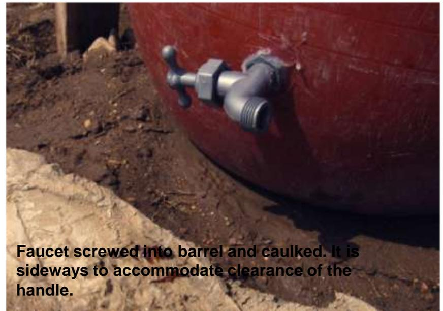
**Faucet screwed into barrel and caulked. It is sideways to accommodate clearance of the handle.**
