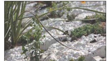
Roof Rock on Madrona Creek Ranch Wellhouse
