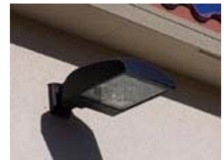
Left: Poorly-designed light. The light from this fixture shoots in all direction (including up).
