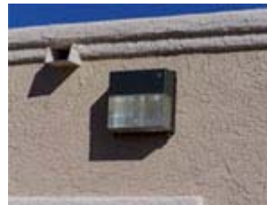
Right: A well-designed full cut-off light. All light is directed down toward the ground.
