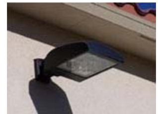
Left: Poorly-designed light. The light from this fixture shoots in all direction (including up).
