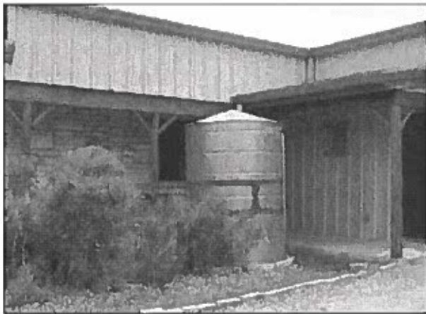
A 2,500 gallon collection tank.
