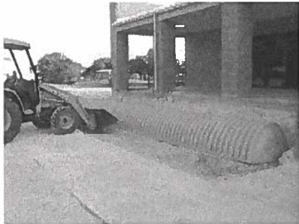
Installation of a soil storage and infiltration system.
