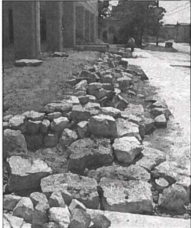
Final landscaping over a soil storage and infiltration system.
